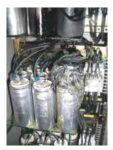
Fig.: Capacitors destroyed by harmonics current
