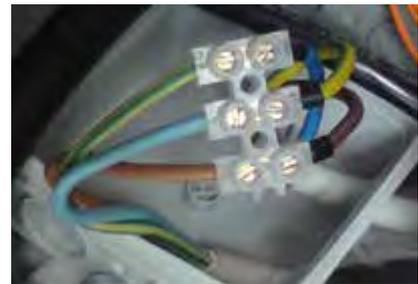
Fig. 7: Here N and PE have been reversed
