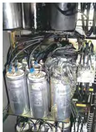
*Fig.: Capacitors destroyed by harmonics current*
